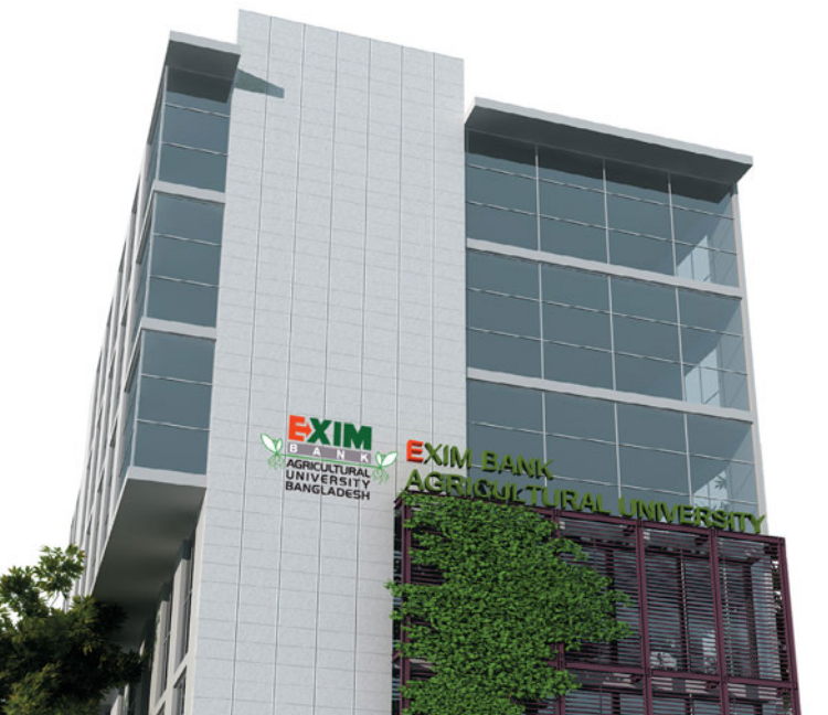
Existing Campus of EXIM Bank Agricultural University Bangladesh at Chapainawabganj
